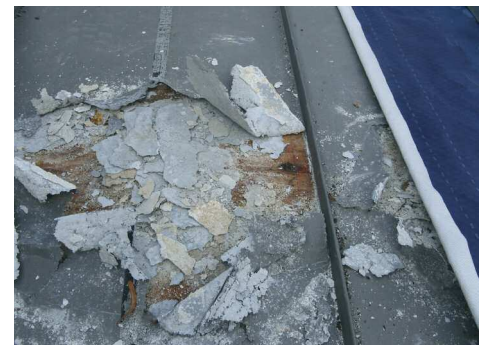
Result of using a hybrid roof
